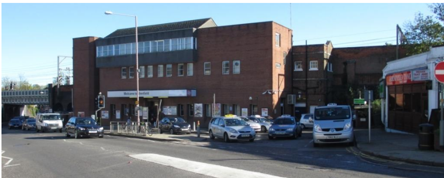
Figure 2-5: Shenfield Station Forecourt Area from southwest perspective
